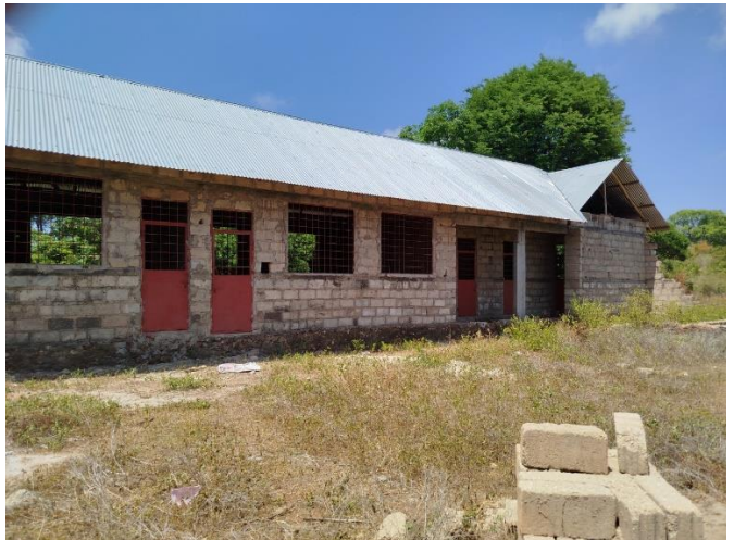
Installatie van deuren en ramen in DARUL KHAIRATI NURSERY SCHOOL (Makunduchi)
